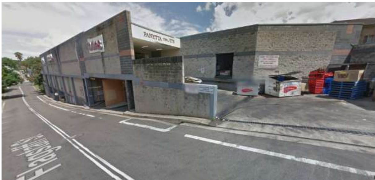
Figure 4 Existing Basement and Loading Dock Access from Flagstaff Street
